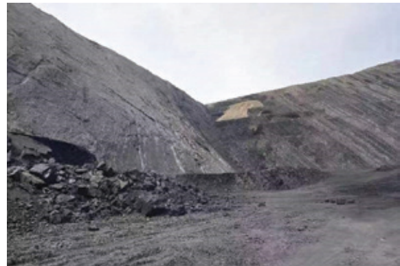
Daily operations of Xingliang Mine
